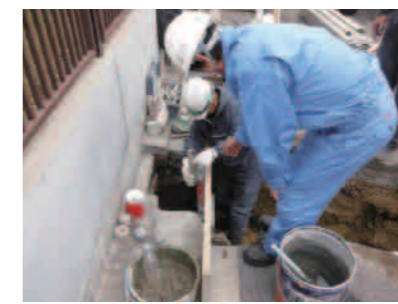
Supervising contractors' work
