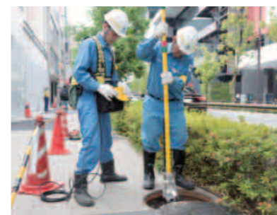
Inspecting sewer pipes (with a zoom camera)
